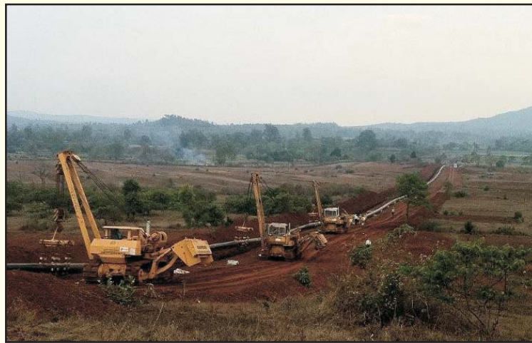
Setting-up a Pipeline System
